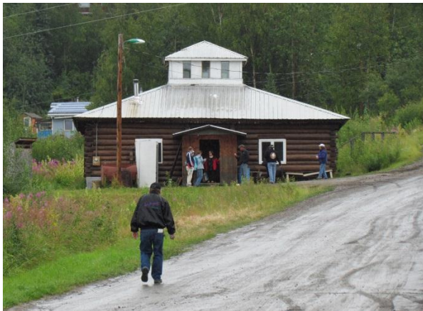
ONAP staff met many residents of the Native Village of Ruby, Alaska, as they gathered at the Community Hall for a meeting on telecom issues. Nestled above the Yukon River, Ruby is in the vast interior of Alaska. While not all the buildings have indoor plumbing, including the Community Hall, the hospitality of the Native Village of Ruby is legendary. The packed meeting covered many areas of the FCC’s regulations and Tribal prerogatives.
