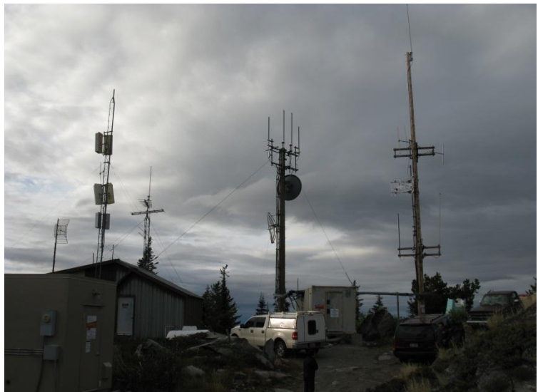
ONAP traveled to the top of 5,747-foot Omak Mountain, located on the Colville Reservation in eastern Washington state, to see towers and communications infrastructure and equipment that serve primarily off-Reservation consumers.
